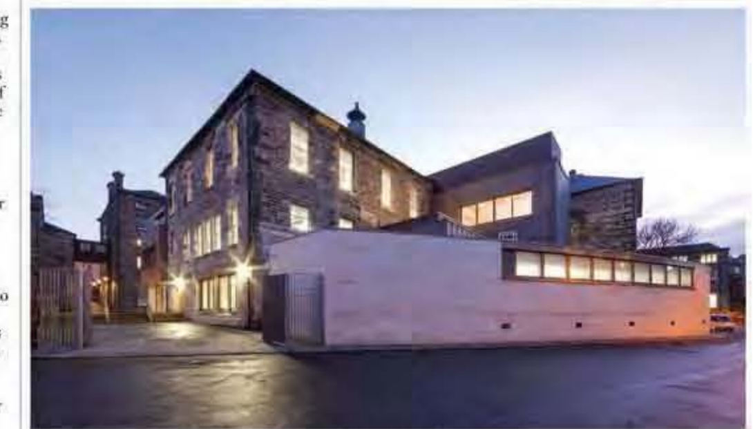
The northern extension presents a masonry wall to the road.
